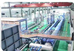
Large-Scale Water Loop Test Facility
